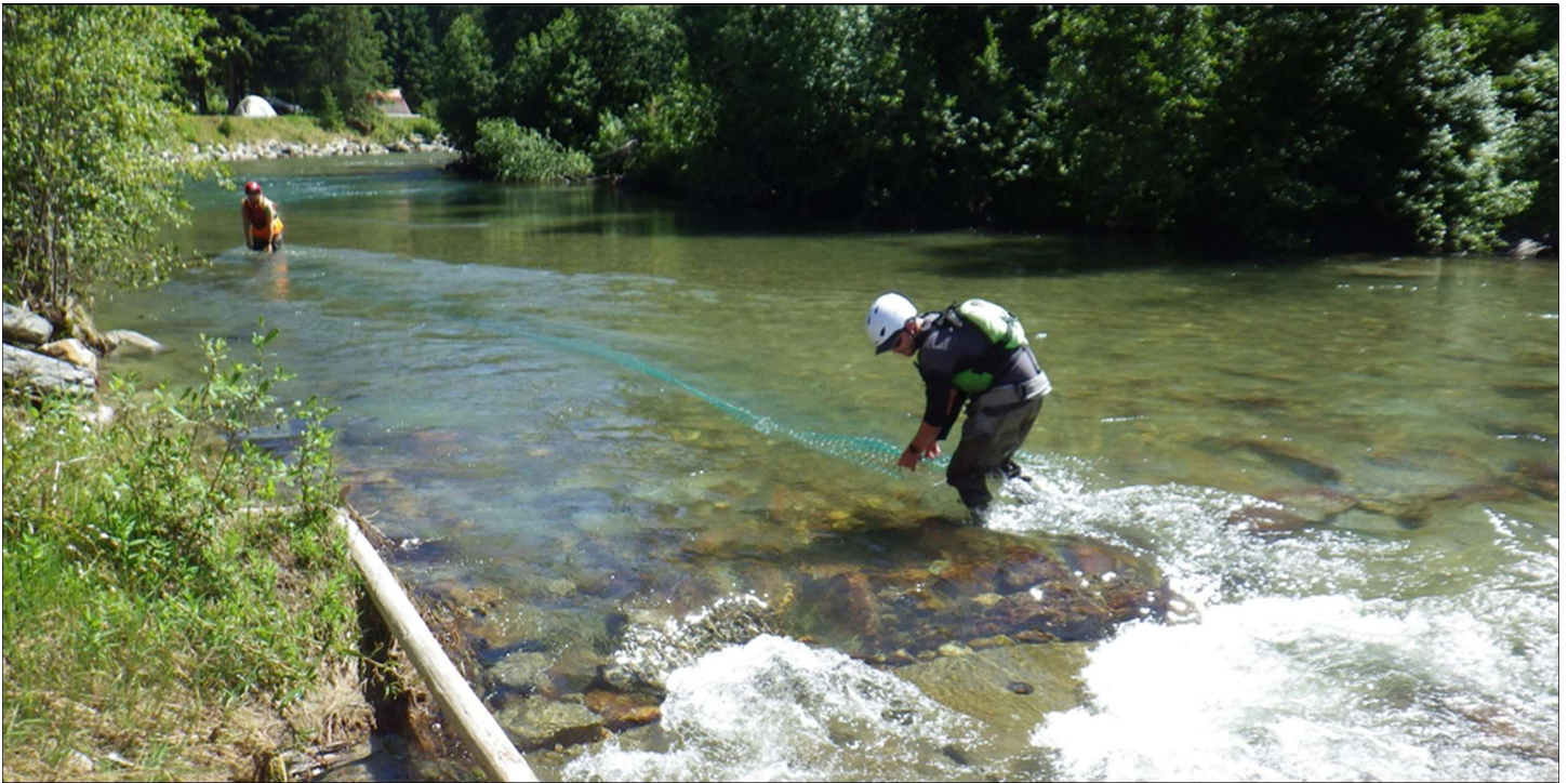
Photo 5. Installation of a spawning deterrent mat roll upstream of the Swift Creek crossing
