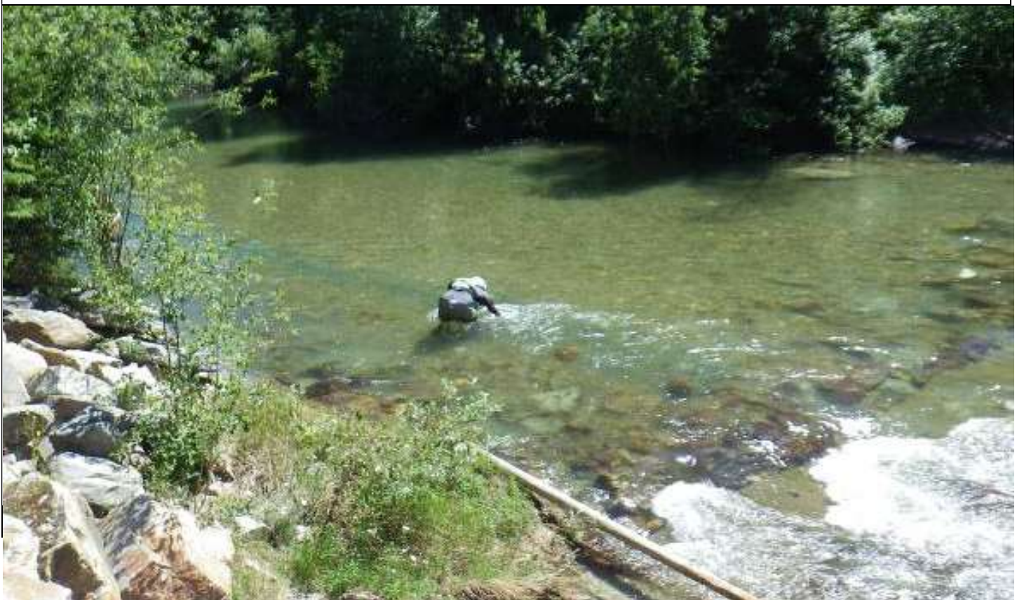
Photo 5. Installation of a spawning deterrent mat roll upstream of the Swift Creek crossing
