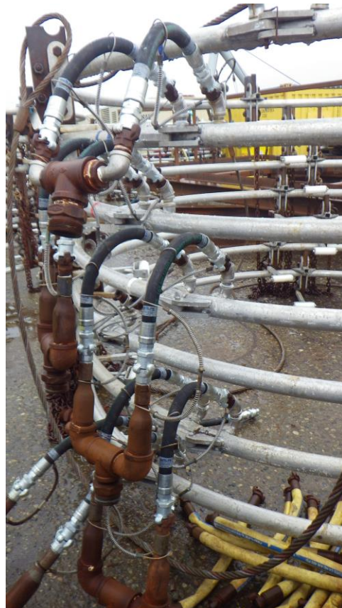
Photo 4. New hoses on bubble curtain rings.
