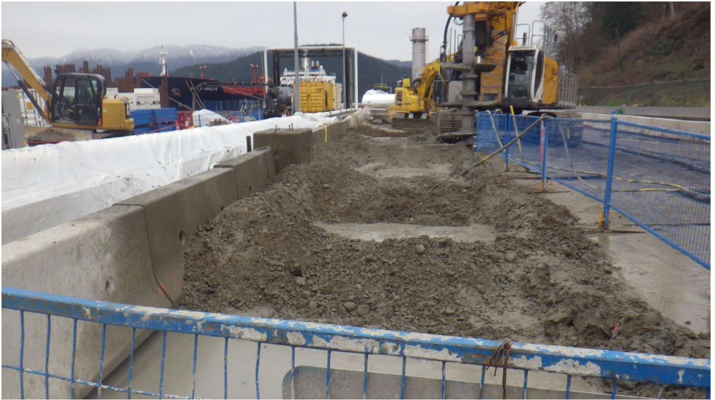
Photo 3. Deep soil mixing columns along foreshore.
