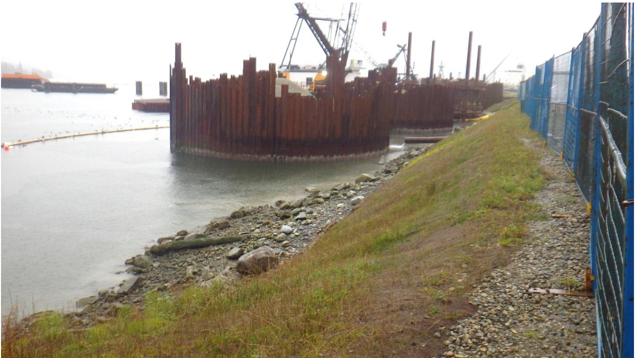
Photo 2. Seeded coco matting has been used to cover areas where riprap has been removed in an effort to reduce erosion.
