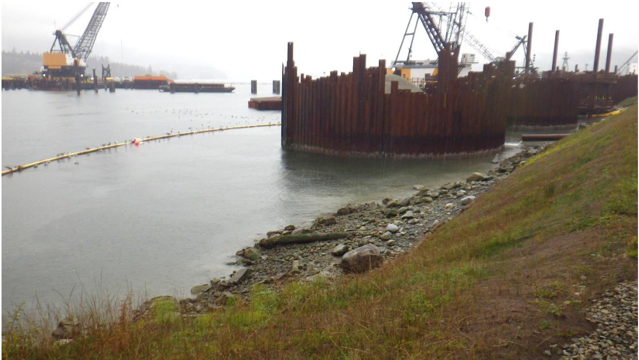
Photo 1. Yellow turbidity curtain installed around the foreshore and sheet pile cells.
