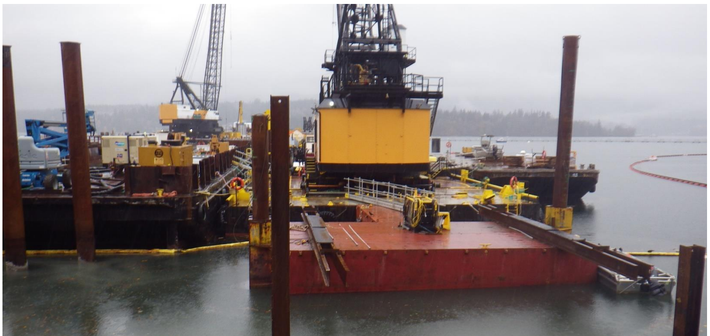
Photo 4. Preparatory works to install the brace frame at sheet pile cell 10.
